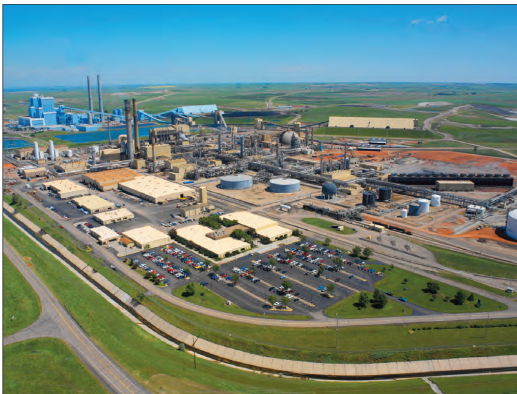
Great Plains Synfuels Plant, North Dakota, USA. A major lignite consumer, since 1984, the plant has been using Lurgi gasifiers to produce SNG and other products. Since 2000, CO 2 from the plant has been captured and piped to Canada for enhanced oil recovery purposes. Around 18,000 tonnes of local lignite is gasified daily (photograph courtesy of Basin electric Power Cooperative)
