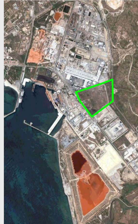
Possible site in Portovesme (CA) industrial zone: plant area 13 ha.
